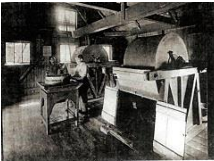
Interior of a mixing house
